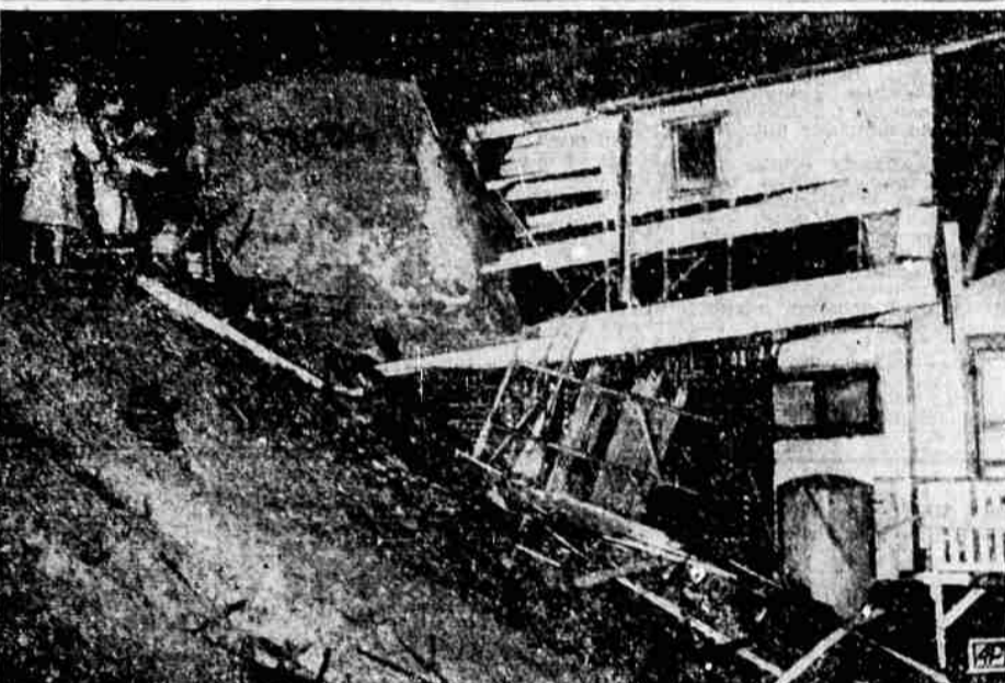
BOULDER WRECKS HOUSE — A five-ton boulder, dislodged by heavy rain from the bluff above this beach house at Malibu, Calif., smashed into the garage which was built above the house.
