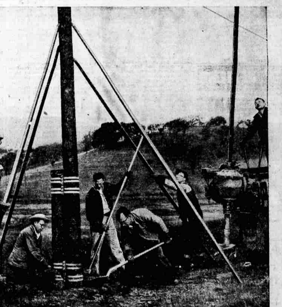
"Pole stubbers" at work: A routine inspection has revealed a pole which shows damage at the ground line. And this crew has been dispatched to reinforce it with a short length. When they're through, it will be as strong as new. And they'll have saved much of the cost of a new pole.
