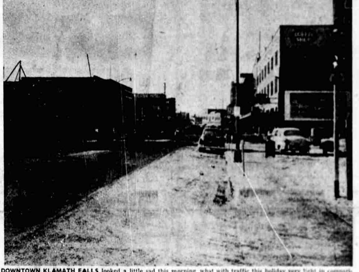
DOWNTOWN KLAMATH FALLS looked a little sad this morning, what with traffic this holiday very light in comparison with the jammed streets of the pre-Christmas days.
