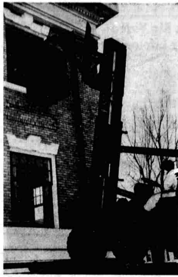
LOWERING THE BOOM with a five-ton safe on the end of its crane is Joe Vincze operating an OK Transfer Co. hoister. In window is John Janssen, foreman, supervising removal of huge safe from city hall offices.
