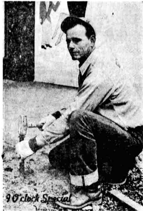
ON THE JOB—R. W. Mitchell, 3136 Cannon, was busy with some curb repair work at Main and 8th this morning. Mitchell is an employee of H. A. Sample, contractor.
