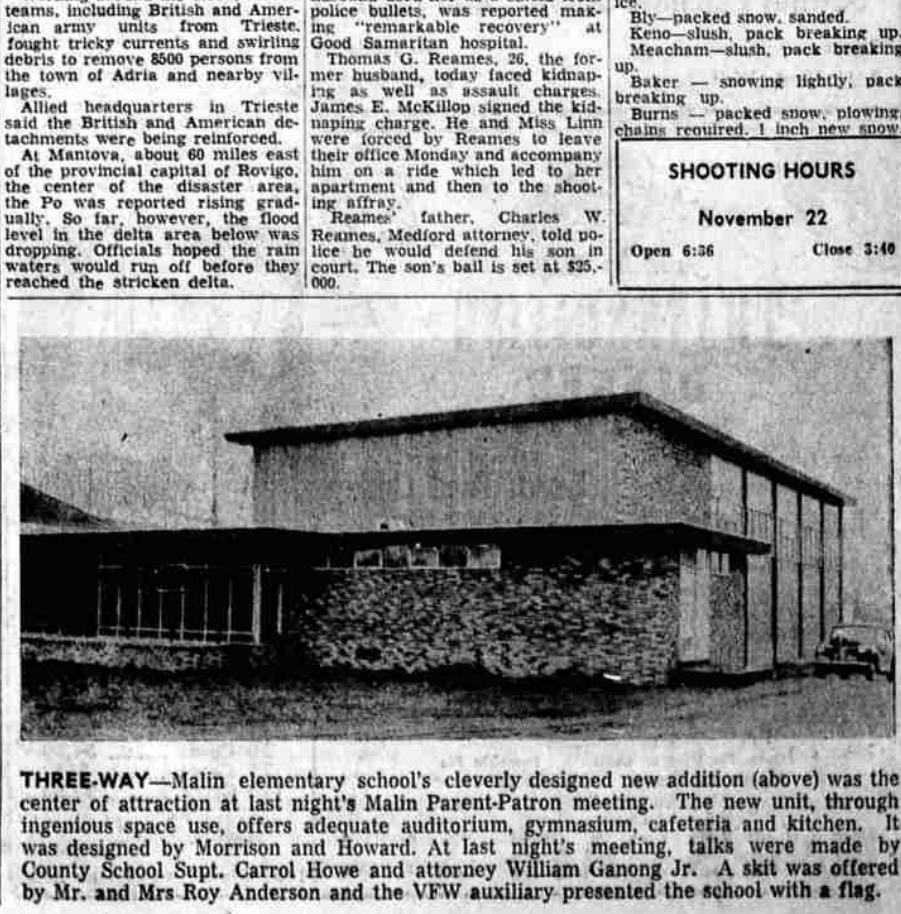
THREEWAY—Malin elementary school's recently designed new addition (above) was the center of attraction at last night's Malin Parent-Patron meeting. The new unit, through ingenious space use, offers adequate auditorium, gymnasium, cafeteria and kitchen. It was designed by Morrison and Howard. At last night's meeting, talks were made by County School Supt. Carrol Howe and attorney William Ganong Jr. A skit was offered by Mr. and Mrs. Roy Anderson and the VFW auxiliary presented the school with a flag.
