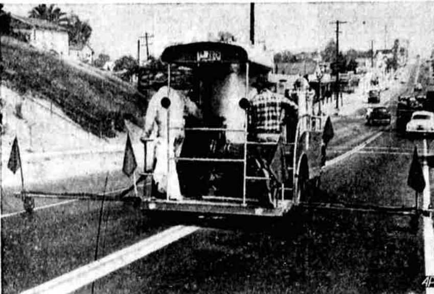
LAYING DOWN THE LINE — Street striping machine invented by a Tacoma, Wash., policeman, lays down double center line and two outside lines in Los Angeles demonstration.
