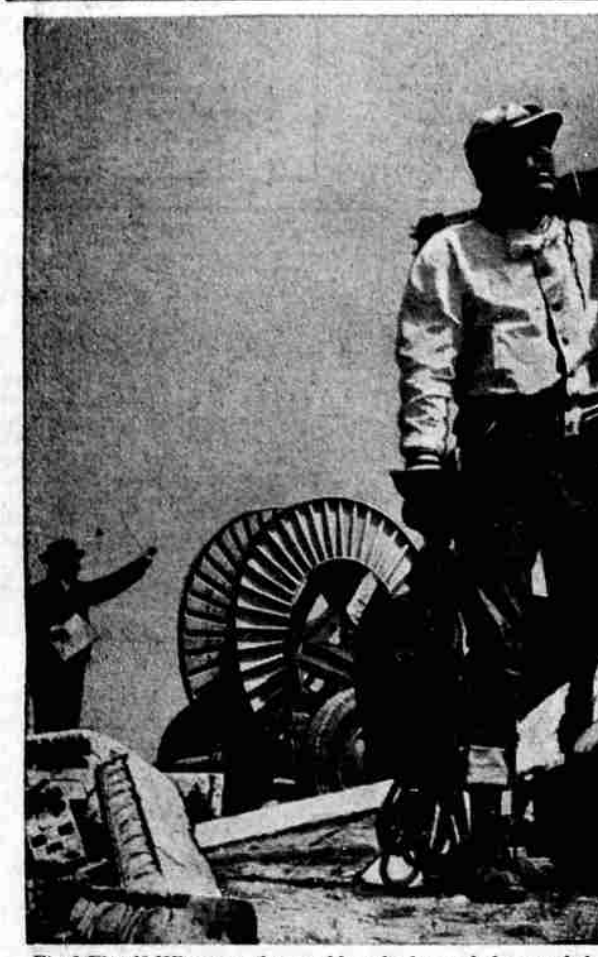
Fire? Flood? Whatever the trouble, telephones help speed the job of rescue and restoration... because we planned ahead.
