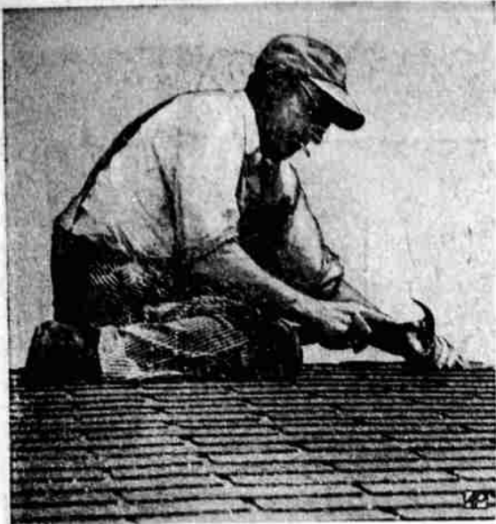
CARPENTER WITHOUT SIGHT —Alex Meuvissen, blind carpenter of Chaska, Minn., lays ridge shingles on house roof depending upon developed senses of touch and hearing.
