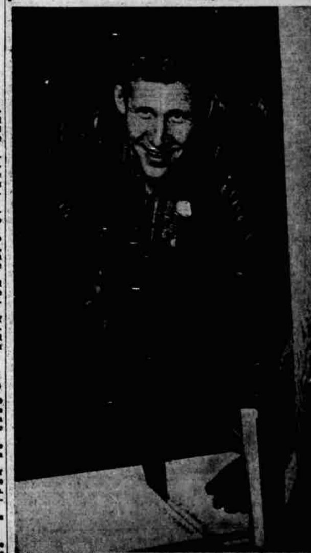
BERT HOGLER is on the business end of a cow as he leads a hand at the First Methodist church where the upper story is being finished for use of Sunday school classes.
