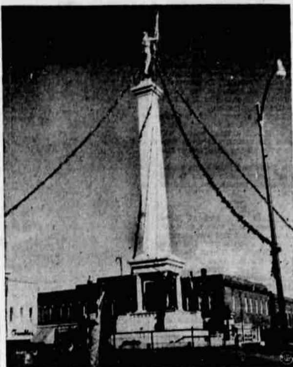
DO TELL! —When archer H. B. Umbaugh of Angola, Ind., shot his arrows into the air, they fell to earth on the other side of Angola's towering monument. In so doing, they solved the town's Christmas decoration problem by carrying over pieces of twine attached to strings of lights. Umbaugh will spend the next few weeks figuring how to get the lights down again without having to climb the statue.
