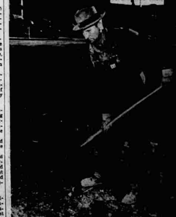
ON THE JOB—John R. Gould hoists a shovelful of dirt on a Main street construction job. It's good weather for building with November days clear and warm.
