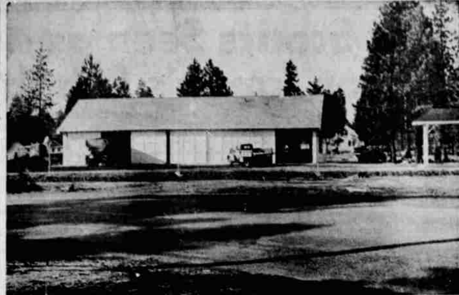
STATE HIGHWAY MAINTENANCE station at Chiloquin, a new project started this summer, is nearing completion and is already in operation. Final touches, such as painting, surrounding fences and lawns are being put in at the unit located at the cutoff junction at the edge of town. This station is one of two new ones being built, the other being at Fort Klamath. The Fort station work is being speeded in hopes of final completion this winter.
