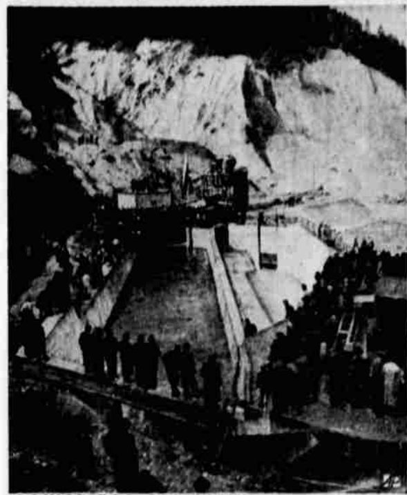
POWER FOR GERMANY — Waters of Riss Creek are dammed to flow through a 4½-mile tunnel under two mountain ranges to Walchen Lake near German Tyrol border. It will increase Lake's power production by 100,000,000 kilowatts a year.
