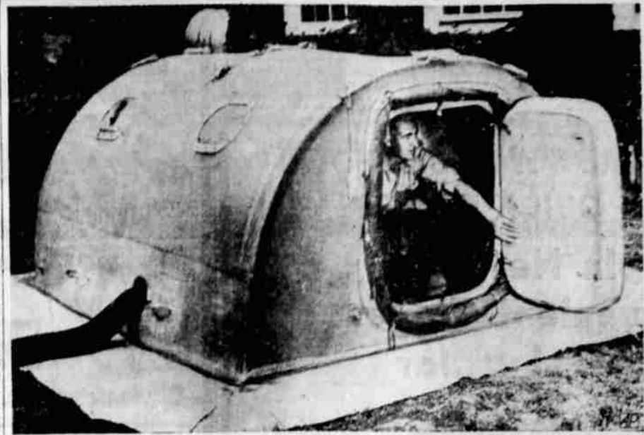
BLOWUP 'QUONSET' HUT —This pneumatic Quonset hut, developed for use in Arctic areas, can be inflated with a simple hand pump in three minutes. The defense department, which released this photograph, says the hut is snow, water and draft proof and has air-tight plexiglass windows; it can support about 500 pounds and can withstand winds of 100 miles an hour. The hose at left is an air duct for ventilation.
