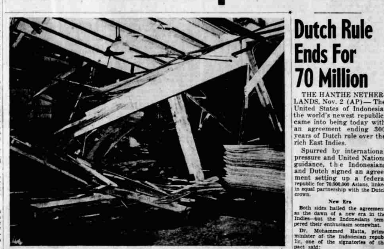
CRUNCH, CRASH AND BANG—A Great Northern box car went the wrong way last night and crashed through the locker room of the Kalpine Plywood plant on the Weed highway. There were no injuries but a sprinkler system was set off and the plant operations halted for the remainder of the night.
