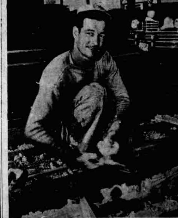
WORKING IN THE FINE sunshine at Esplanade and Main is a fine summer job for Irvin Smith, cement finisher, who is polishing up the island where a traffic signal will soon be installed to regulate the heavy flow of town moving vehicles.
