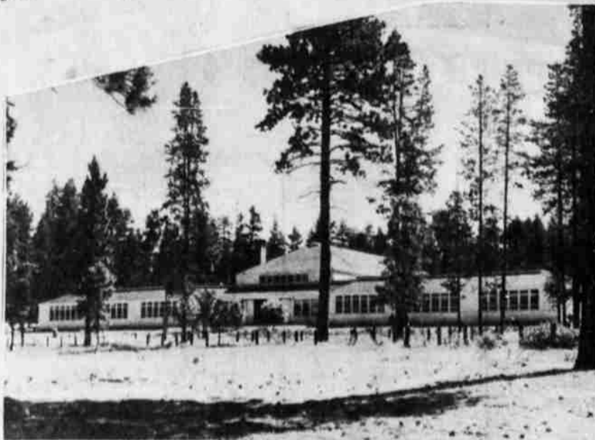
Gilchrist school has made walking easier and more delightful with new floor covering from Calhoun's.
