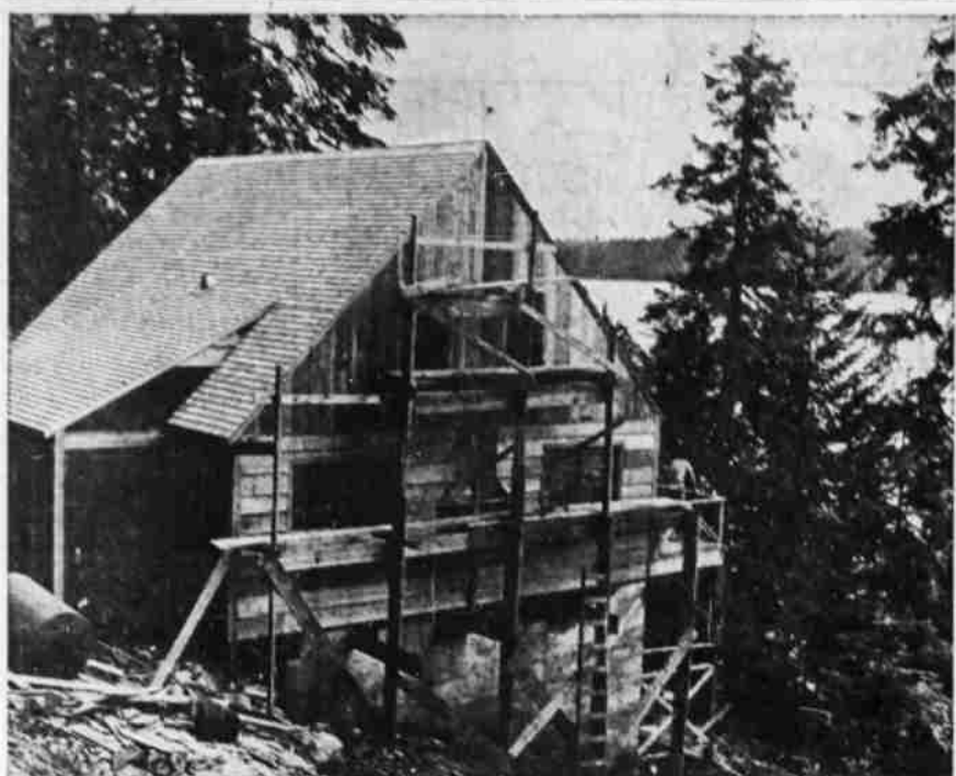
REBUILT STRUCTURE —One of the newly built cabins at the Lake o' the Woods is that which belongs to George Bratton Sr. The cabin was entirely rebuilt after the original was razed by snow and wind last winter. The seven-room cabin, which is on the west side of the lake, is almost completed now.
