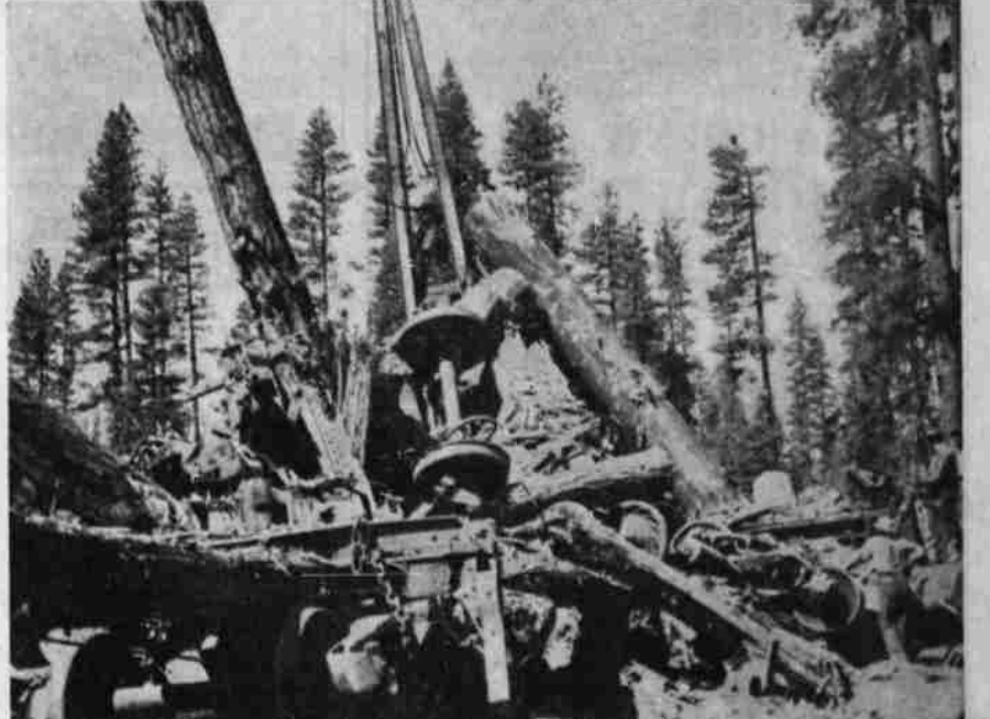
CAMP 4 WRECKAGE —A twisted mass of steel and timber resulted when a string of 24 cars loaded with logs broke loose at 4 a. m. Thursday morning near Weyerhaeuser Camp 4 and came to a stop in jumbled wreckage after rolling six miles. The loaded cars were set out above the loading ramp the day before, preparatory to shipping. It was not known what caused the cars to start the wild roll down the six-mile incline. Several of the cars were almost completely demolished and 11 of them spilled their loads. No one was injured.
