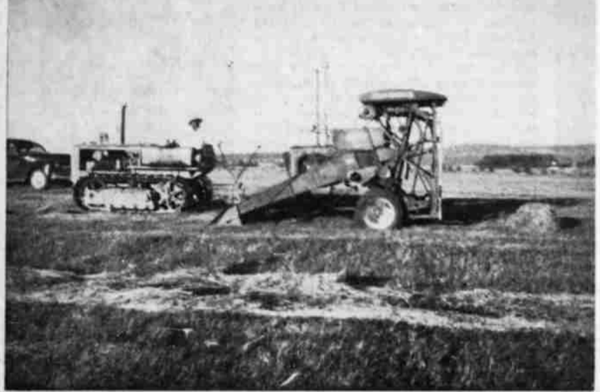
ROTO-BALER WORKS PRACTICALLY ALONE—Only one man on a tractor can bale a field of hay in short order making the bales round instead of square with the use of a machine recently introduced in the Klamath basin. Melvin Fiegi, Poe valley rancher, is the man on the tractor.
