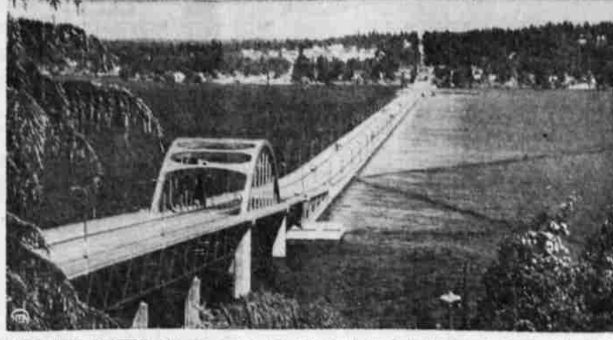
CONNECTING SEATTLE with the eastern shore of Puget Sound is the unique floating Lake Washington bridge. This view is looking from Seattle toward Mercer Island, the other terminus of the floating structure.
