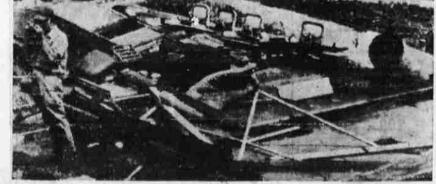
OKINAWA TYPHOON DAMAGE —Twisted wreckage is all that remains of the Guest House at headquarters, Ryukus command on Okinawa, following a devastating typhoon which struck the Pacific island. Sixteen Americans were injured, one child was killed and millions of dollars of property damage inflicted by the storm which lashed the island with winds up to 150 miles an hour.
