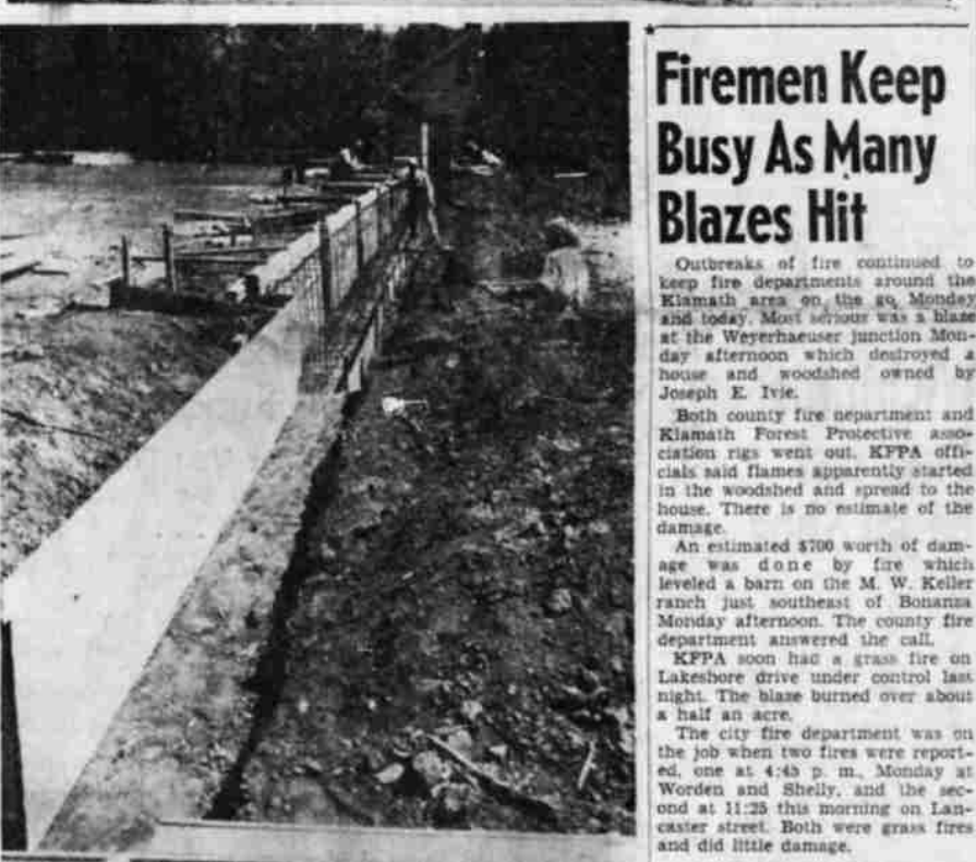
EIGHTH STREET CONSTRUCTION—North Eighth street is now a scene of busy construction activity, as these pictures demonstrate. Upper view shows work proceeding on a wing on St. Paul's Episcopal church, Eighth and Jefferson, which will house a minister's study and parish house. Below, pouring proceeds on a wall, part of the major project between Sacred Heart church and academy, where a new recreation center and parish hall will be finished this year.
