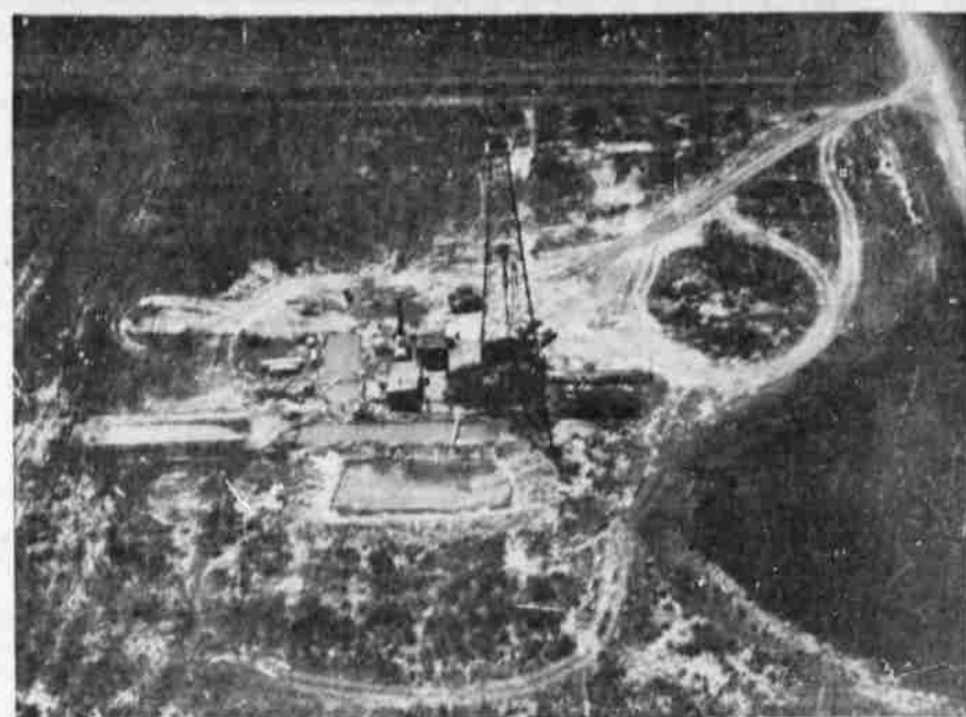
4000 FEET DOWN —And still going. This picture shows the oil derrick of the United Company of Oregon at Burns, where encouraging signs have been located.
