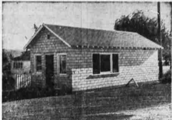
MODERN RANCH OFFICE—This neat, compact building is part of the modern ranch setup on the Poe valley holdings of Don Liskey, Klamath county rancher.
