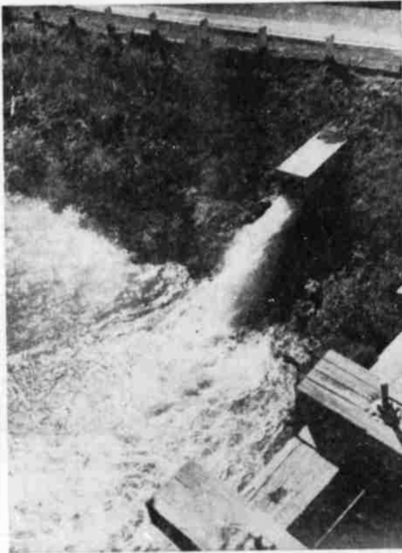
EXCESS WATER—What would be overflow from irrigation ditches when they are running at capacity, is let out through a spillway. This spillway lets the water out into Lost river, thus acting as a safety valve and saving banks from caving under the tremendous pressure of water. The spillway is located just below the big flume at the Poe valley cutoff from Olene.
