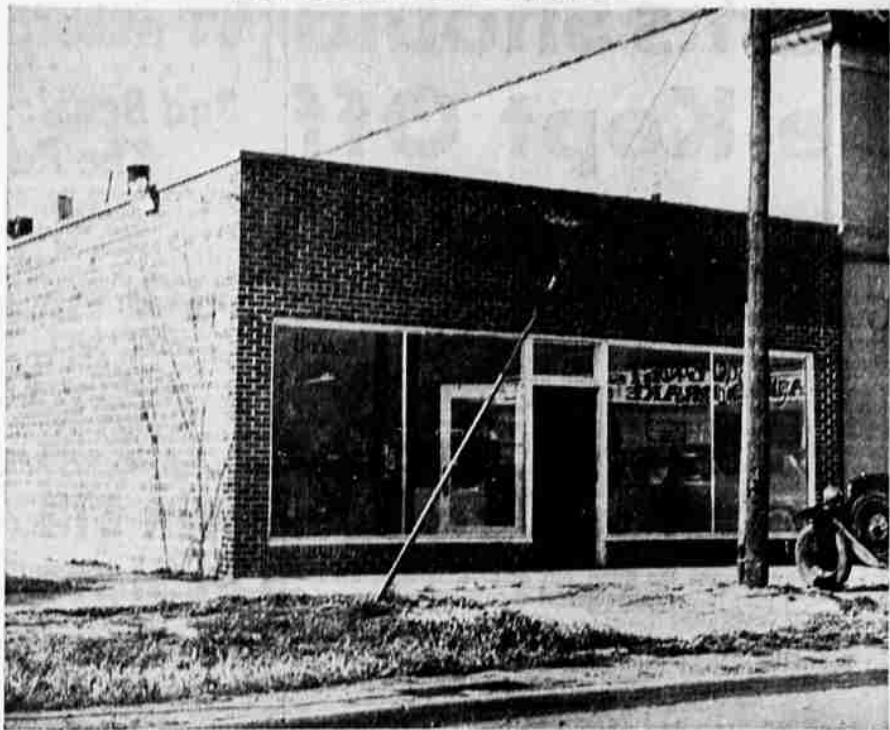
This new business building has just been completed at 1717 Main street, representing further development in the business district just east of the underpass. This structure was erected to house Bob's Self-Service laundry, operated by Bob Friesen, and was constructed by the Friesen family.
