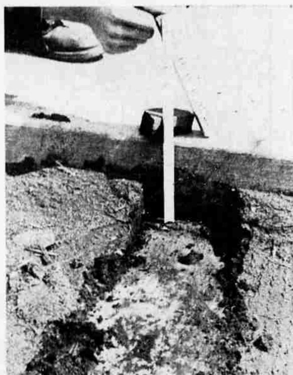
Three inches of caked dirt against curb on Walnut, between 7th and 8th, near post office.
