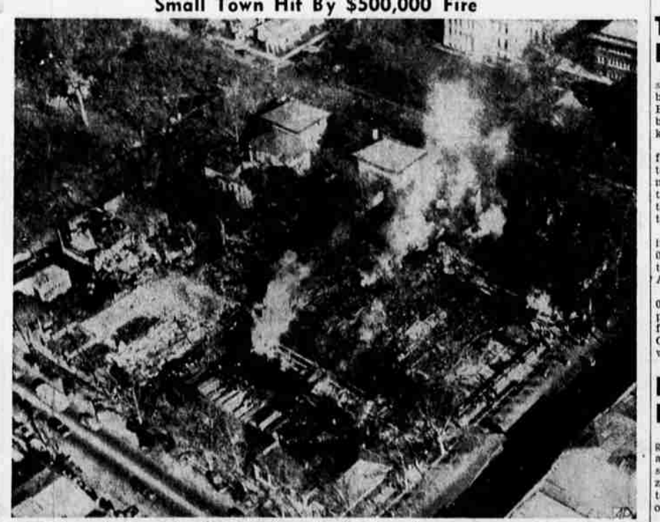
This is an air view of the $500,000 pre-dawn fire which blazed in a lumber yard and farm, Yuma, Calif., and leaped before a strong wind to destroy the yard, a church, plumber's store and four two-story dwellings. No one was injured, but firemen from nearby Yuba City joined a four-hour battle to stop the flames.
