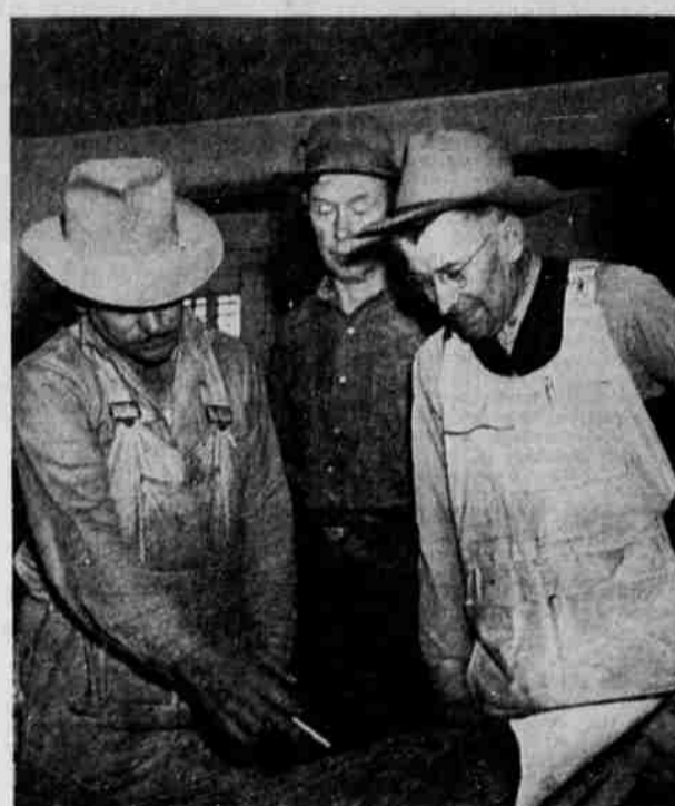
The Klamath Falls carpenters' union came to the rescue this week with an offer to donate labor to the Teen-Age Center's remodeling project. Doors were being yanked out and enlarged, partitions were being removed and the building donated for the teen-agers' use by Mr. and Mrs. R. P. Olliver at 228 N. 8th. From left are four who donated their services: Guy Malotte, Earl Goddings, D. McGilivray and C. E. Robinson. All except McGilivray are carpenters, and McGilivray was just there to help out. Several more carpenters were on the job today.
