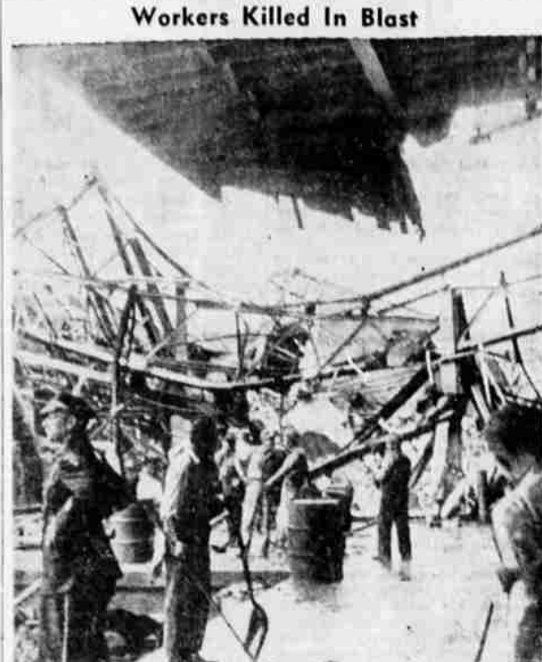
Workers Killed In Blast An explosion which wrecked the engine test building of International Harvester company plant in Louisville, Ky., took the lives of at least seven workmen. Twenty-six persons were injured and twenty-five others trapped in the debris. The blast occurred as the night shift was leaving and the day shift reporting. —AP wirephoto
