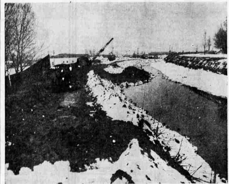
Tons of earth are being moved by the U. S. bureau of reclamation along the canal adjoining Klamath Union high school property in an effort to correct seepage conditions on the main government ditch. This picture shows dragline operations where a trench is to be excavated and then backfilled with compacted material.
