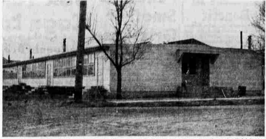
This is one of the buildings constructed from old Jap buildings at Camp Newell on the Tulelake high school grounds. Instruction in general farm management will be given here under the veterans vocational agricultural program.
