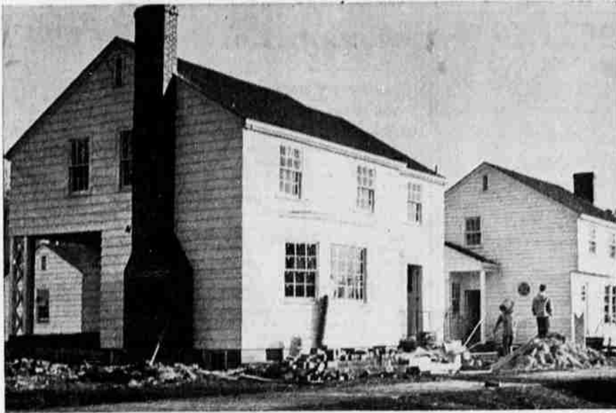
These two-story, white-painted houses located on Eldorado between Fremont and Manzanita, follow the general styling of the New England Cape Cod houses and have full basements.
