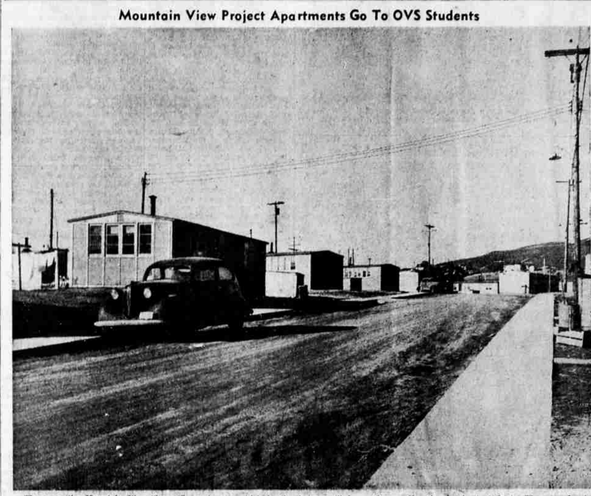
These are the Mountain View "boxcar" apartments which in the future will house Oregon Vocational school students. They are located at the end of Main street and this picture was taken looking down Chiloquin avenue. The apartments are of frame and composition construction and were designed as temporary dwellings three years ago.
