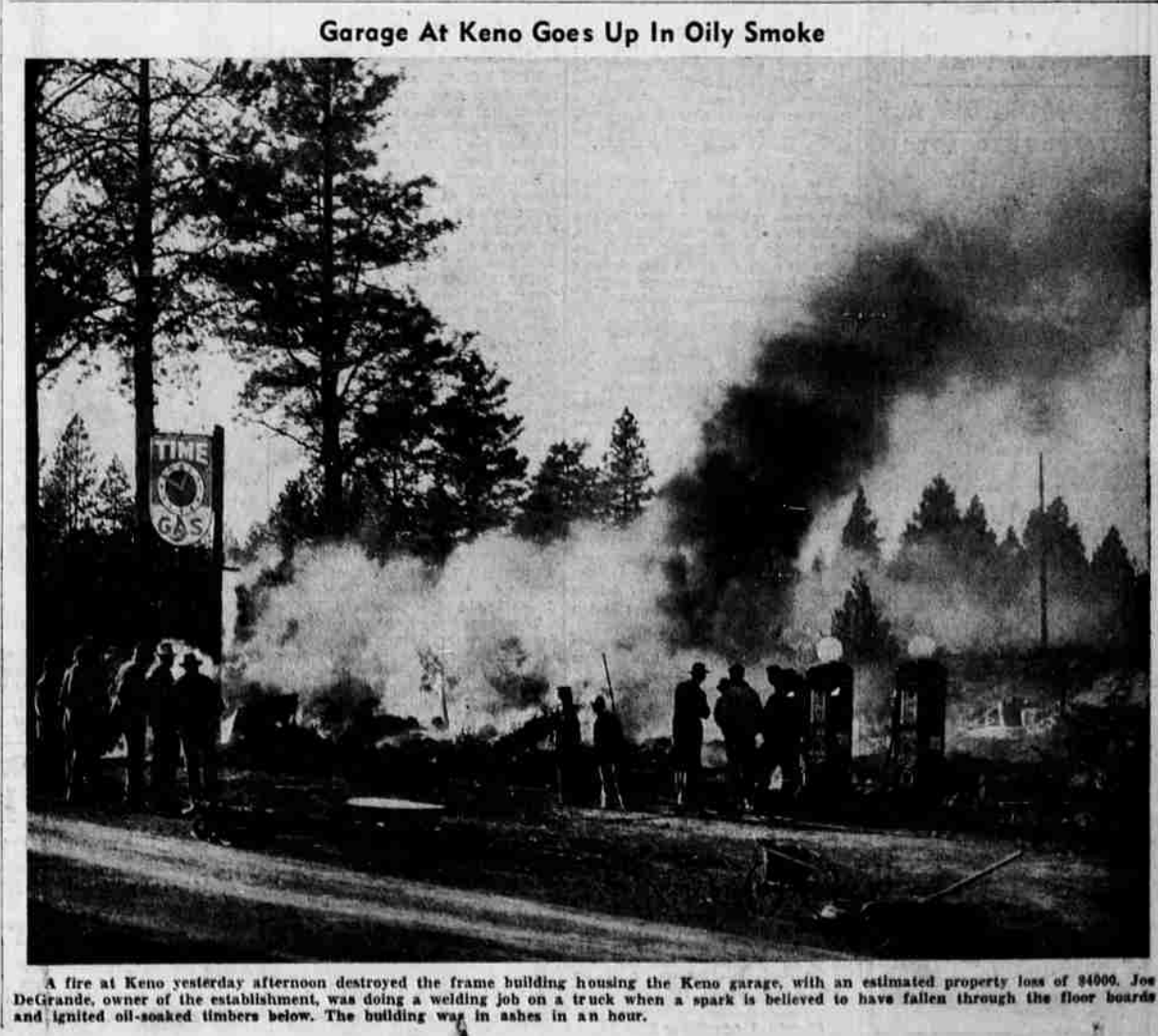
A fire at Keno yesterday afternoon destroyed the frame building housing the Keno garage, with an estimated property loss of $4000. Joe DeGrande, owner of the establishment, was doing a welding job on a truck when a spark is believed to have fallen through the floor boards and ignited oil-soaked timbers below. The building was in ashes in an hour.
