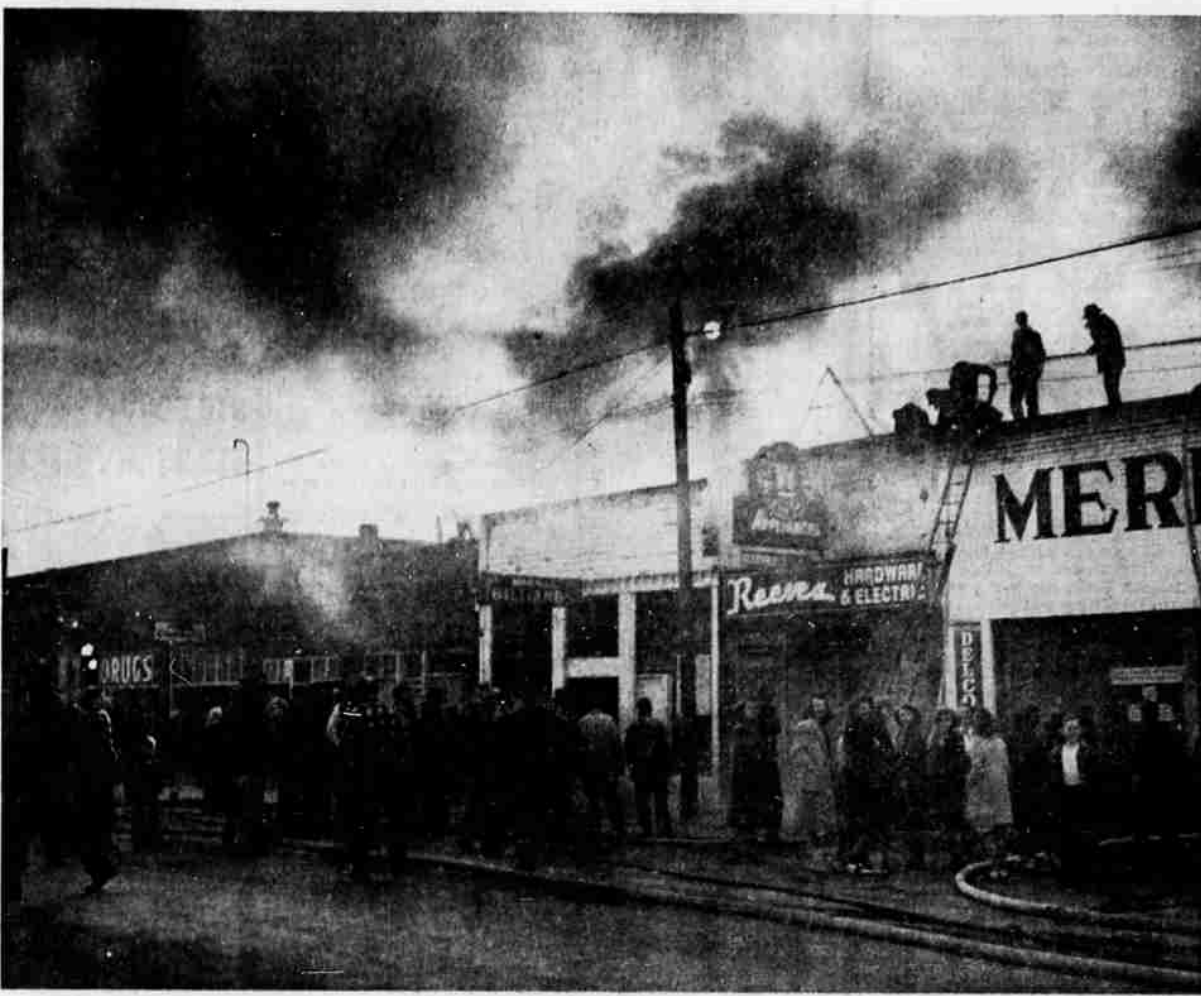
TWO MERRILL BUILDINGS BURNED OUT —Two buildings in the center of the Merrill business section were virtually destroyed by a fire of unexplained origin early this morning, a fire which was kept from spreading by walls of brick structures on either side of the burned spots. Most of the damage was done in the Merrill Billiards, which was gutted, but the Reeves hardware and electrical service also received severe fire, water and smoke damage. Two trucks of the Merrill volunteer fire department and one truck from Malin fought the blaze for two hours before it was put out. The fire was believed to have started in the pool hall and was discovered when Darrell King, one of the owners, came to open for business at 7:15 a. m.
