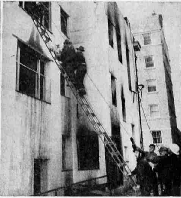
DISASTER —A body is removed from the Evans apartment building after the disastrous fire of February 16.
