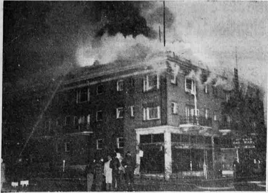
FIRE! —Disaster and violent death ran tragically through the news of 1947. The early morning picture above shows firemen playing water on the burning Evans building, 10th and Main, on February 16. Five lost their lives in this blaze.
