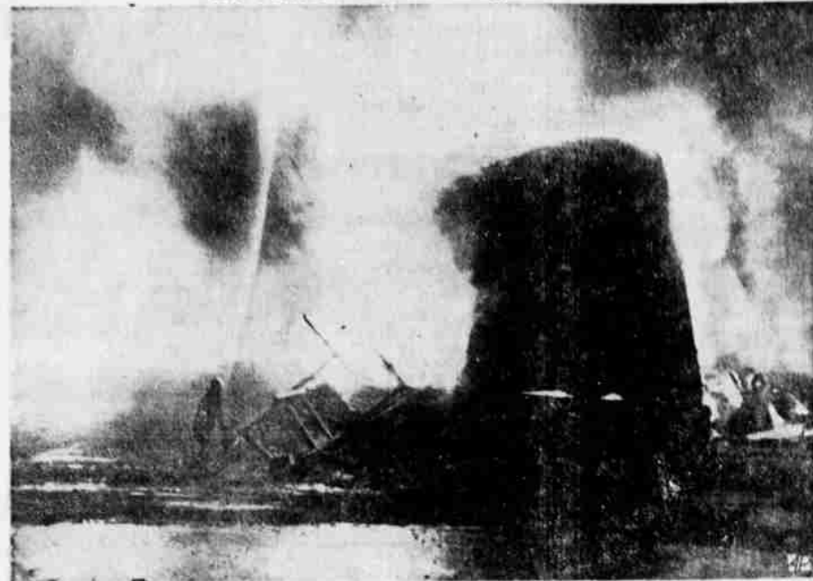
An inferno of flames rises from two oil tanks which caught fire in an explosion in the Signal Hill oil field at Long Beach, Calif. Firemen succeeded in preventing the flames from spreading to other tanks and oil wells.
