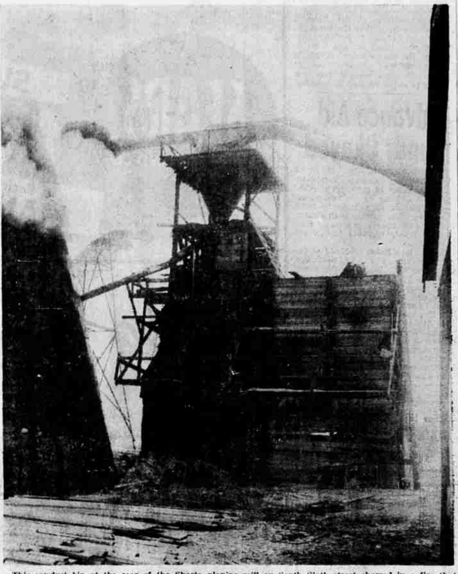
This sawdust bin at the rear of the Shasta planing mill on South Sixth street charred in a fire that broke out there about 7 o'clock last night. City and county firemen quickly checked the blaze, and damage was slight, as this picture taken this morning shows. The fire was in the center of an industrial district.
