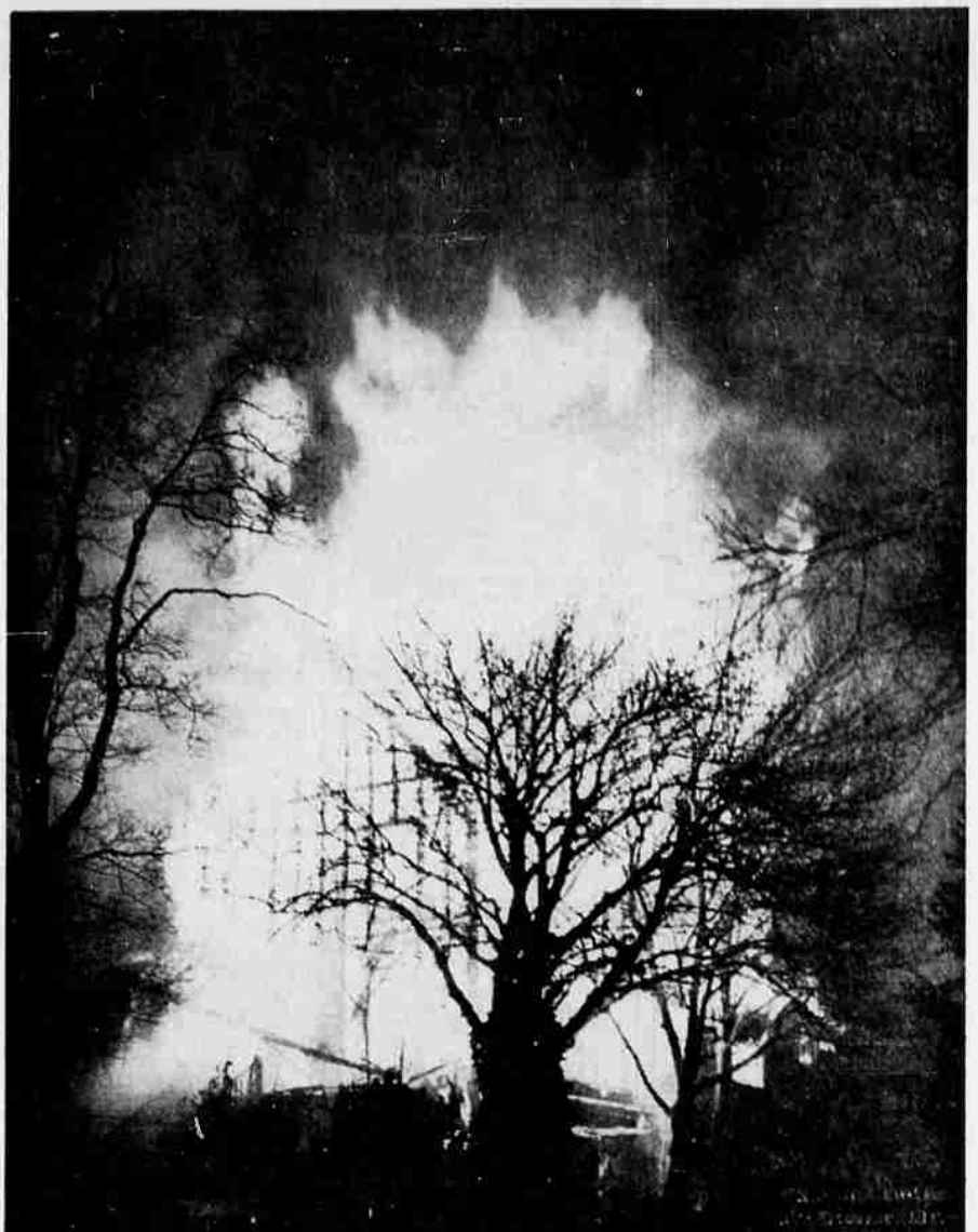
This is the flaming structure of the Harry O. Brown home in Dunsmuir destroyed by fire early Tuesday morning, taking the life of Mrs. Brown and causing serious burns to her husband, pioneer Dunsmuir resident. This place is a landmark in that section of town, located on the highway one mile north of the Sacramento river bridge.
