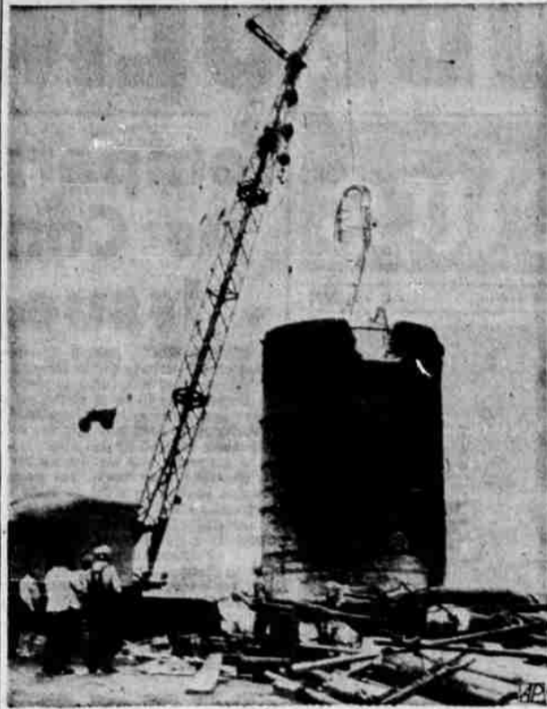
In the gray mist of morning a mobile crane at Everett, Mass., pulls from an active-gas-fume chimney a portion of the wreckage of a small plane that crashed into the structure as it sought a place to land in foggy darkness. Aboard the plane, and killed, were four persons, an industrialist, owner of the ship, his two daughters, and the pilot. —AP wirephoto.
