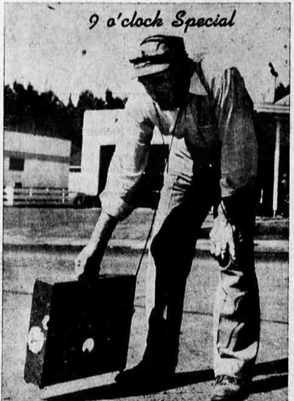
The man with the earphones and "suitcase" is Glenn Bowen, superintendent of the California Oregon Power company water department. The "suitcase" is an amazing device called a pipe locator, which operates on the same principle as a mine detector in locating water mains and valves beneath the ground.
