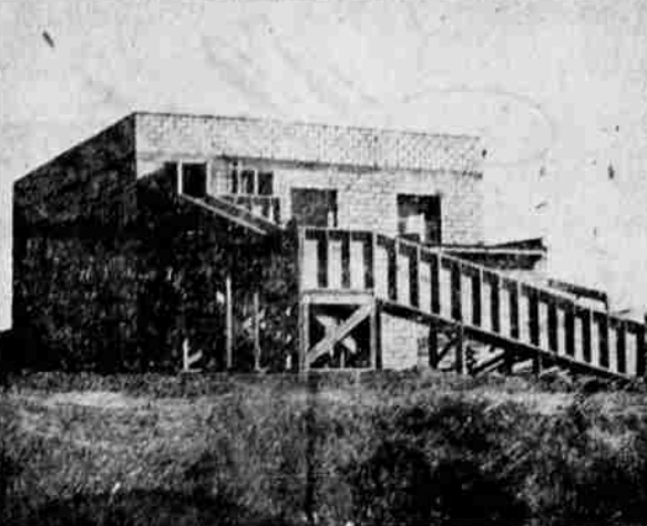
This new slaughter house going up just past Mac's store on the Merrill highway is being built of pumice tile by Tom Barry and Dale Moore, who expect to start operation in a few weeks. Hogs will be driven up the outdoor ramp and shot when they reach the top. Just like shooting fish in a barrel.
