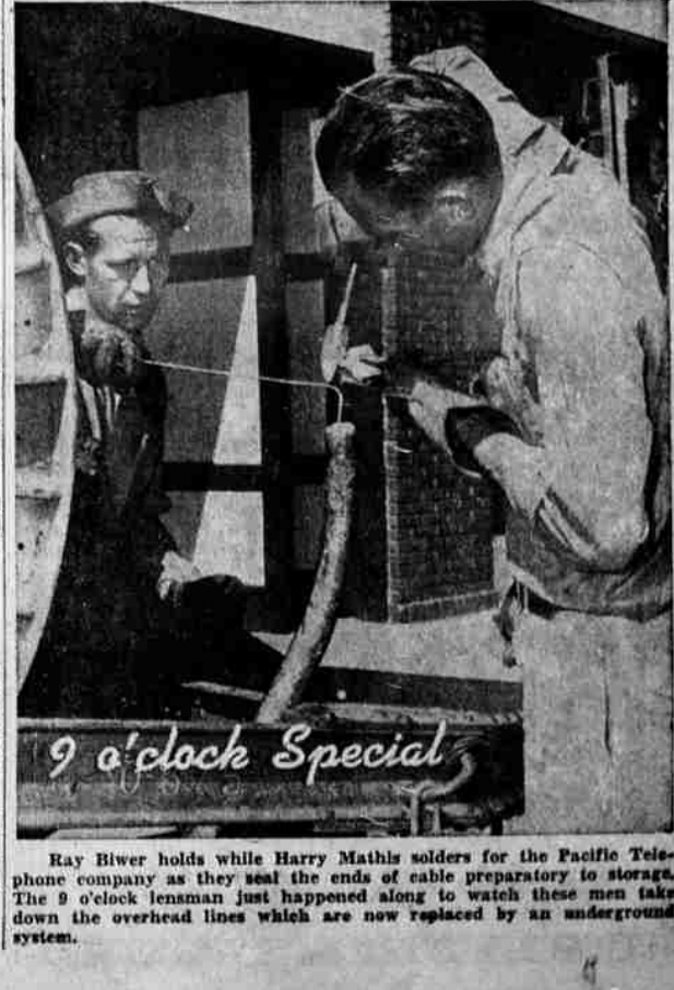
Ray River holds while Harry Mathis solders for the Pacific Telephone company as they seal the ends of cable preparatory to storage. The 9 o'clock lineman just happened along to watch these men take down the overhead lines which are now replaced by an underground system.
