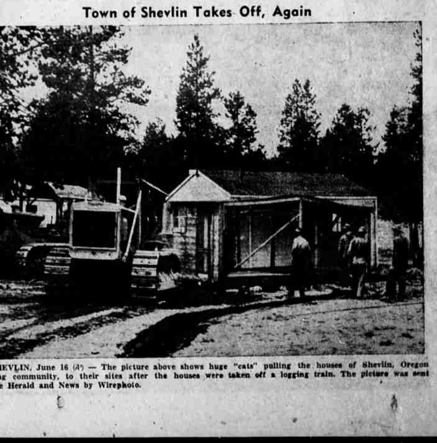
SHEVLIN, June 16 (AP) — The picture above shows huge "cats" pulling the houses of Shevlin, Oregon logging community, to their sites after the houses were taken off a logging train. The picture was sent to the Herald and News by Wirephoto.
