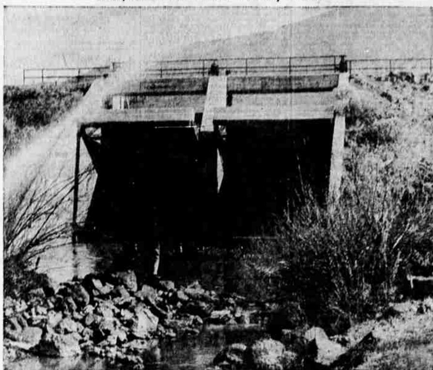
A boy and his dog contemplate the cool water trickling over Malone dam on Lost river in Langell valley. This dam, built by the U. S. bureau of reclamation in 1923, is 32 feet high, 515 feet long and is used to raise the water in Lost river which is supplied from Clear Lake reservoir, and to divert it to the west canal for irrigating farm lands west of Langell valley.
