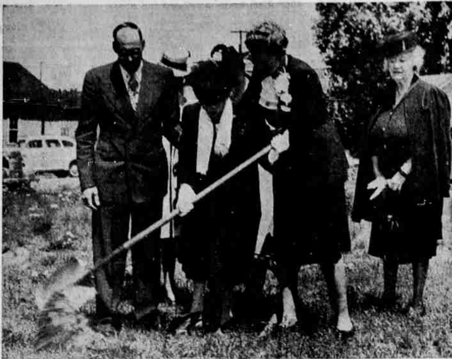
Mrs. Laura Chamberlain, only living charter member of the Immanuel Baptist church, turned the first spadeful of ground in ceremonies last Sunday with construction of a new building slated to begin immediately at the site, N. 11th and High. Left to right: Rev. Charles Sundstrom, pastor, Mrs. Chamberlain, Mrs. Lucille Binns and Mrs. Fred Ohlemeyer, long time members of the church.
