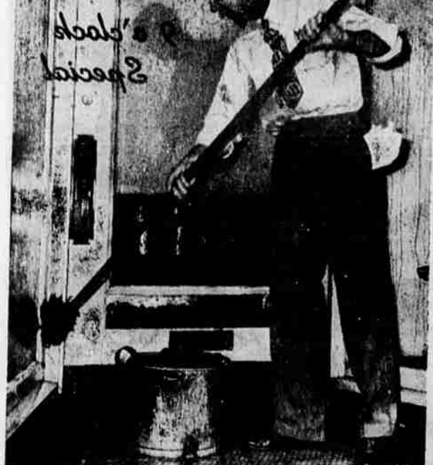
This is a common sight up and down Main street, washing off the windows in preparation for the day's business. The 9 o'clock Special picture man snapped Marvin Furlow welding the brush at Dick Reeder's this morning.
