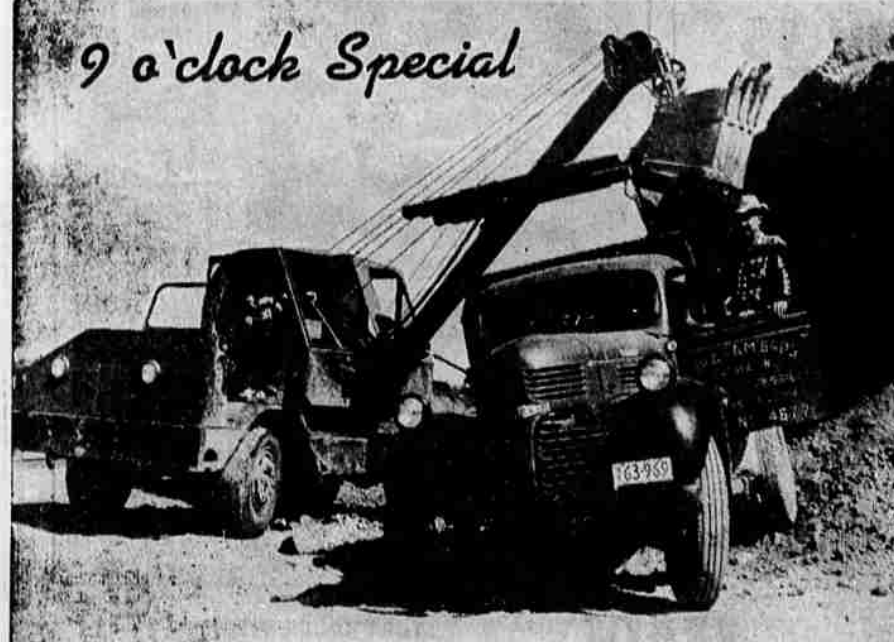
Yards of dirt either out of the mouth of the scoop into the Graham Brothers truck as the 9 o'clock lensman witnessed the above scene at that hour this morning. Stepping into his truck is Herbert Graham, one of the brothers.
