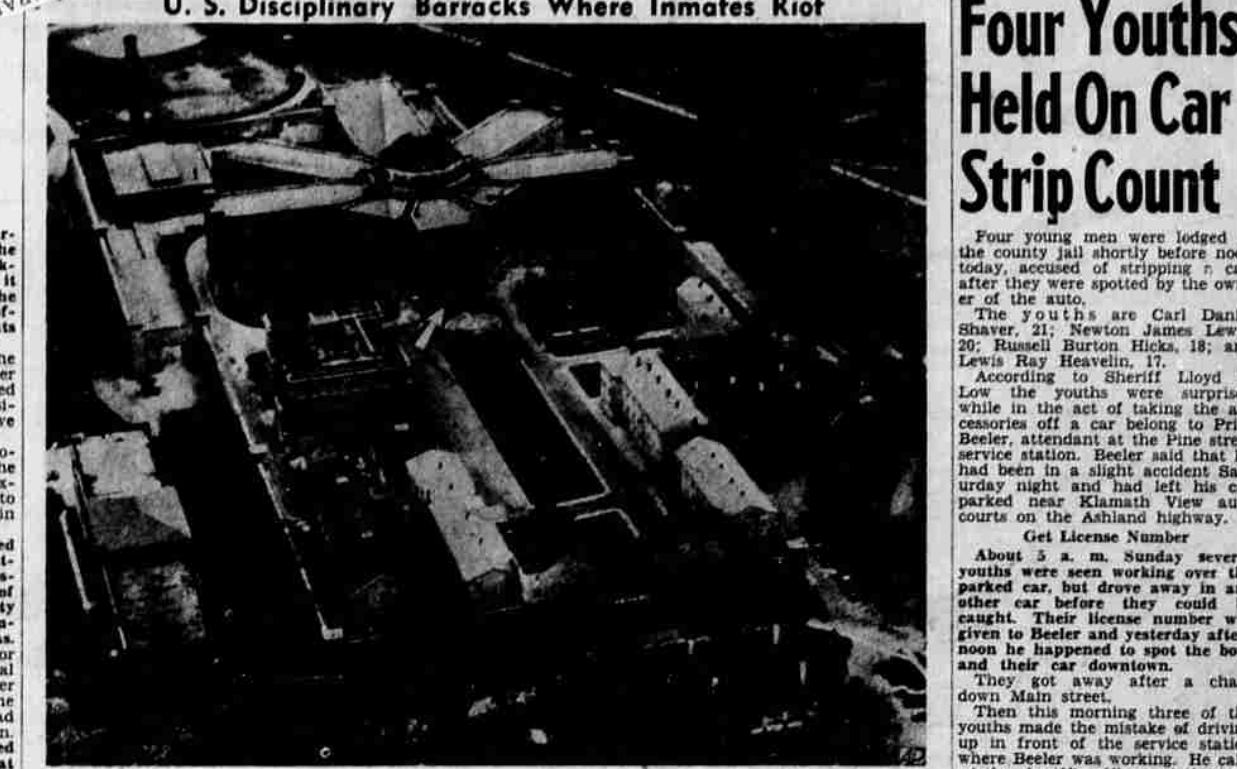
This is an aerial view of the U. S. disciplinary barracks, Fort Leavenworth, Kas., where guards quelled a riot by about 800 prisoners. One inmate was dead and seven others injured in the disturbances. Main entrance through wall is in center foreground. Arrow indicates men around door to building entering cell block area. Picture made as rioting was in progress.
